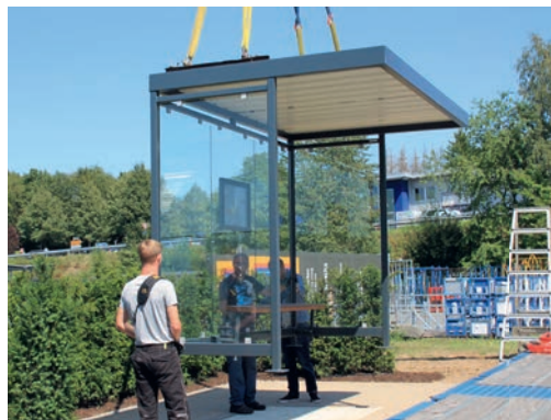
Installation in one piece: Installation of a completely welded and assembled public transport stop by our logistics and assembly team.
