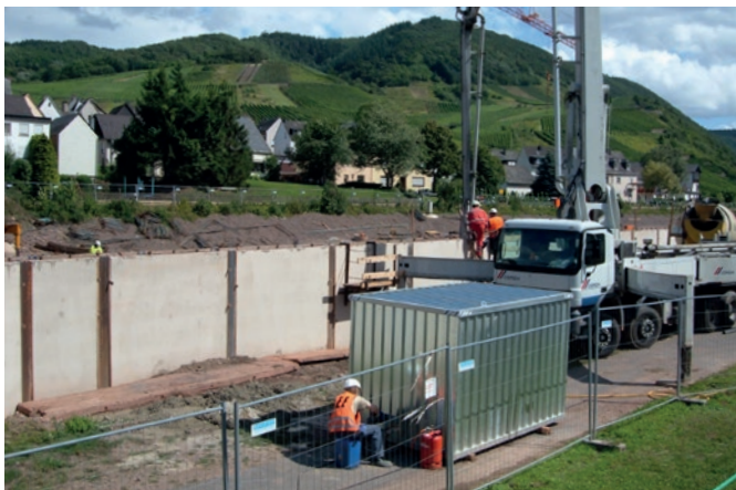
SC3000 on a construction site
