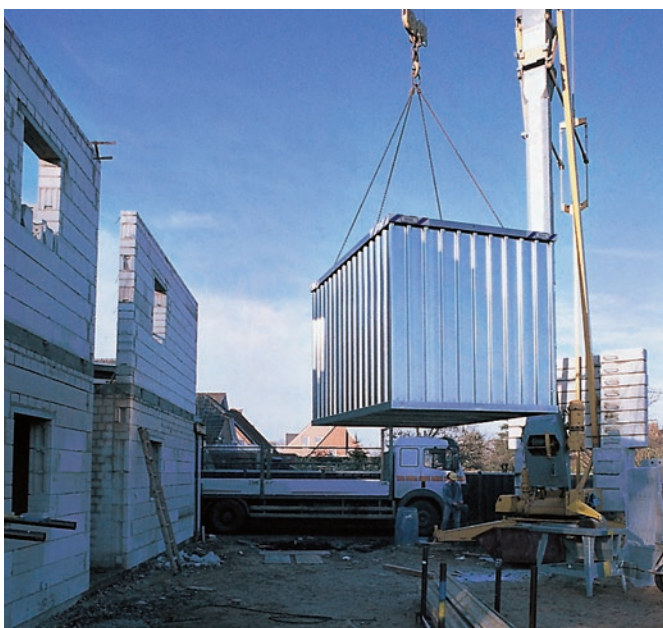
With 4 standard jack rings, up to 3 tons can be lifted by crane
