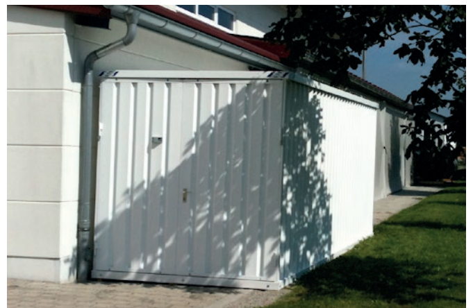
SC3000-6x2SZ as storage space
