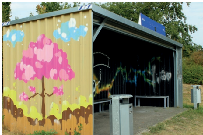
Shelter at the Skatepark Emsdetten/Germany
